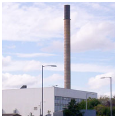
CHP Boiler House at Edinburgh's Western General Hospital
