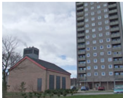
Boiler House and one of the 4 blocks in Stockethill served by the scheme.
